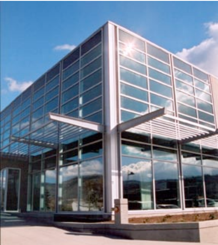
Kamloops Centre for Water Quality | LEED-NC Gold Kamloops, British Columbia
