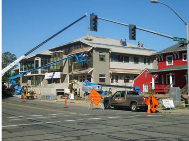
Solar panel installation on Washington Public Utilities Director's Headquarters (Courtesy of Mountain Construction)
