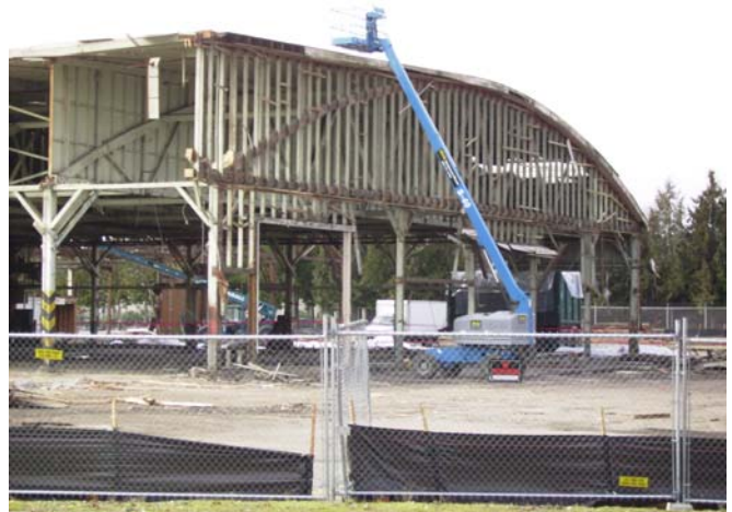
Port of Olympia East Bay Warehouse Demolition by KMB Design Development
