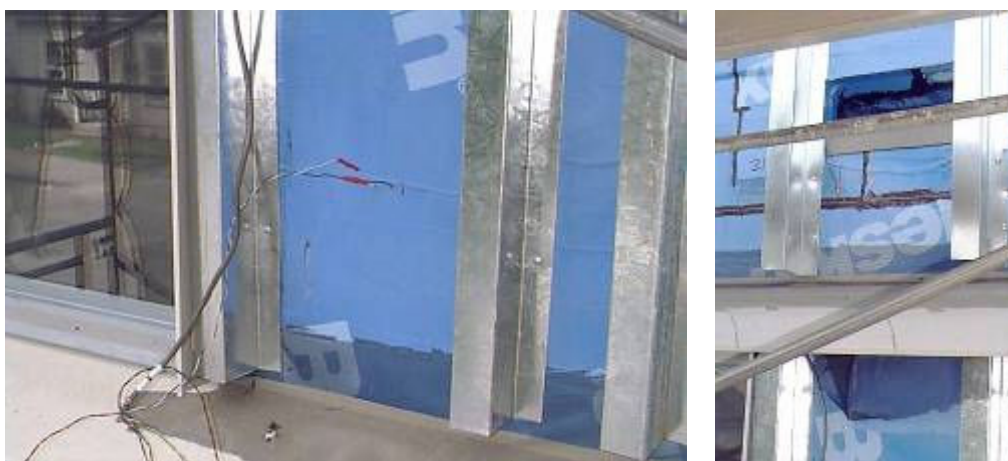
Figure 1-7: Building 3 – Air Barrier Membrane over Gypsum Sheathing
