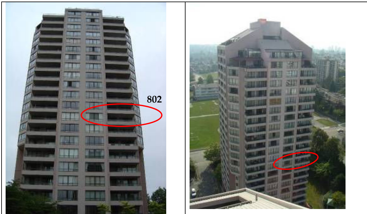
Figure 1-11: Building A – Overview of South Elevation
