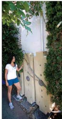
Allison Ashcroft shows off the rainwater collection system at her Rebecca Street home.
