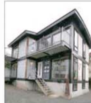
RAY SMITH, TIMES COLONIST Zigloo Domestic demonstrates new use for old shipping containers.
