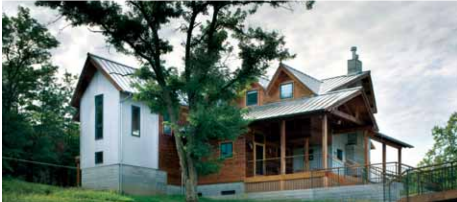
THE NET-ZERO ENERGY GREEN DIRT RESIDENCE MEETS NEARLY EVERY REQUIREMENT OF A LIVING BUILDING, FEATURING RE-PURPOSED BUILDING MATERIALS WHILE MEETING THE HIGHEST STANDARDS FOR ENERGY EFFICIENCY AND CARBON REDUCTIONS. PHOTO COPYRIGHT © BOB GREENSPAN.
