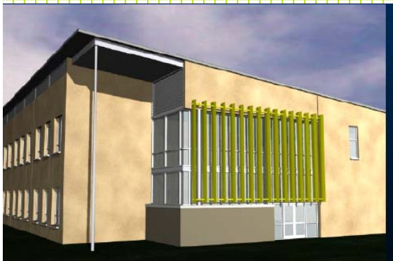
Vertical sunscreens at east and west windows of The Dalles Middle School provide shade in late afternoon, while still providing access to views. Graphic courtesy of Boora Architects
