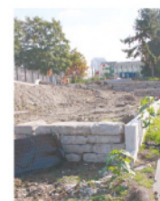
Cascade Park under construction - completion scheduled for late 2004
