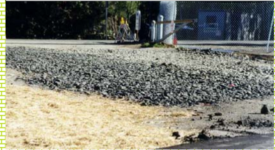
Best practices on the site, such as this rock construction entrance prevented silt from being tracked onto roads and back into nearby waterways, a major concern on the Sakai project which was sited adjacent to a salmon stream.
