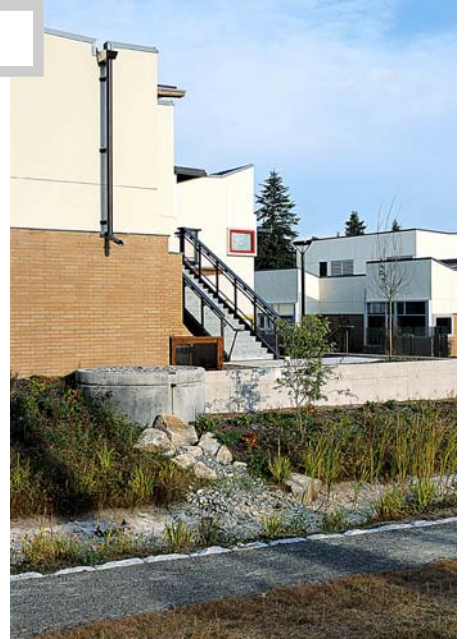
Terrace Park School’s major roof forms are pitched toward their centers in a “butterfly” form designed to capture rainwater and direct it to where it is most visible. The rain falls onto the roof, flows into scuppers, and then into concrete cisterns. Overflow from the cisterns pours into swales, that slowly release water into the site’s drainage system. Wetland plants in the swales treat the water by filtering out toxins and sediment before the water reaches the nearby creek.
